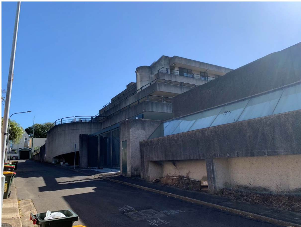
Ferry Lane elevation of MRC Building (south)
