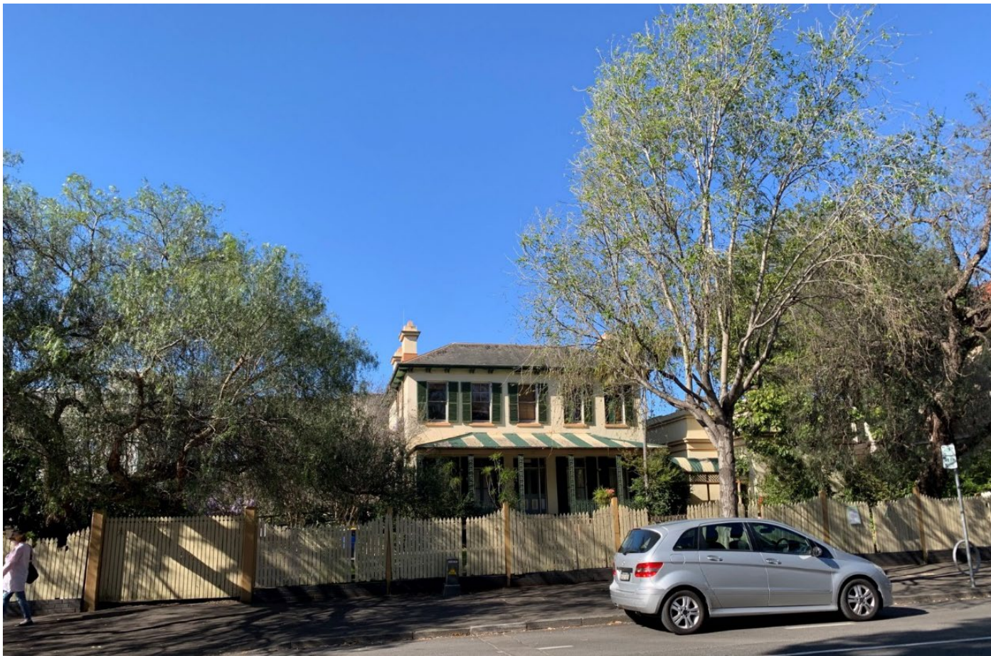
Bidura House viewed from Glebe Point Road
